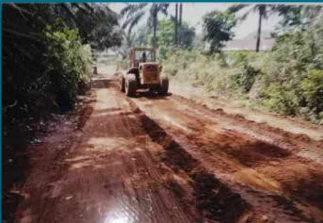
The Roads rehabilitation and maintenance in some parts of Obiuno Community...
