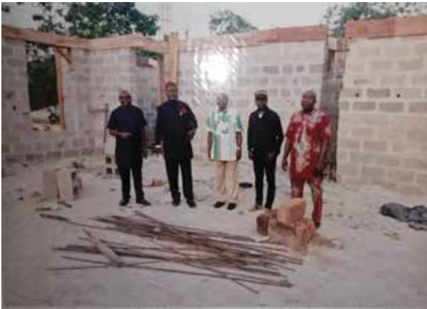
Just before the FIRST decking in July 2019
